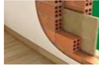
Figure 23 Double Walls: It Consists of Two Layers of Bricks, Between Which There Is A Space for Thermal and Acoustic Insulation [NAGHAM HAIDER, (2021)].
