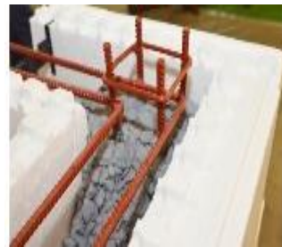
Figure 21 ICF Insulating Concrete Walls [NAGHAM HAIDER, (2021)].
