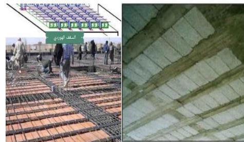
Figure 25 Hollow Block Slab [MUHAMMAD, (2020)].
