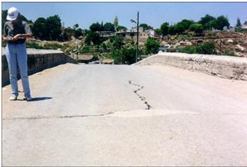
Figure 3: Damages occurred in superstructure of the Misis Bridge during the 1998 Adana-Ceyhan earthquake (Ural et al. 2008)
