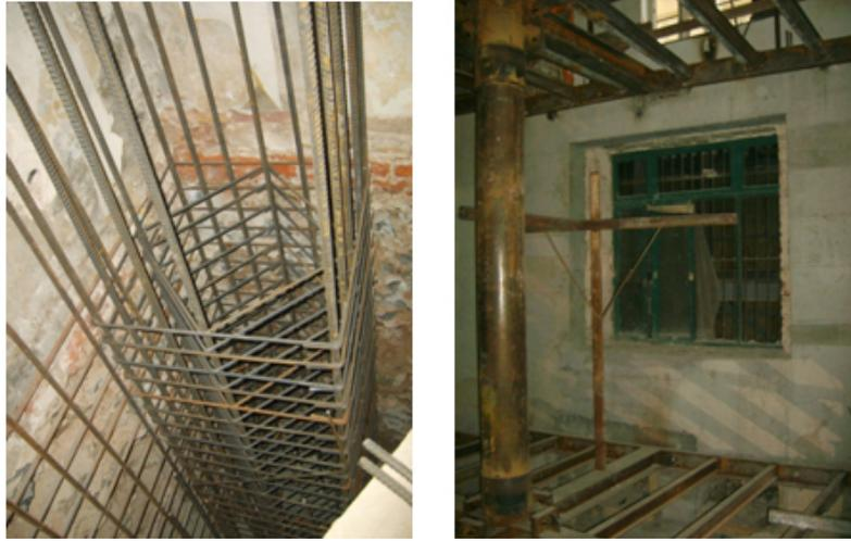
Figure 14. Reinforced concrete columns and shear walls
