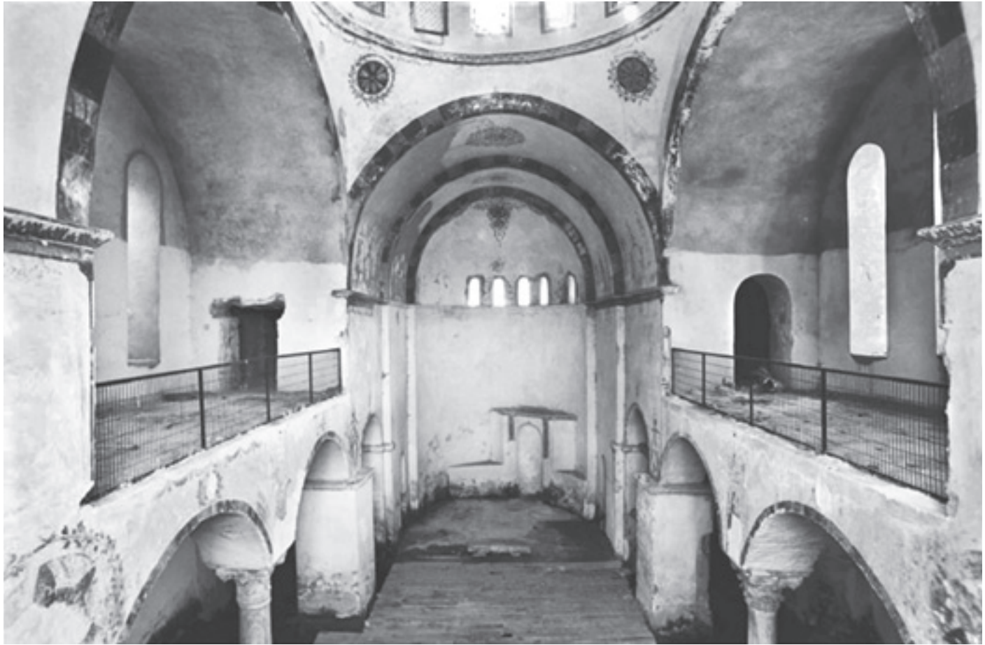
Fig. 13. The Church of Hagia Sophia in Bizye (Vize) (after: Bauer, Klein, Hagia Sophia in Bizye , fig. 5)
