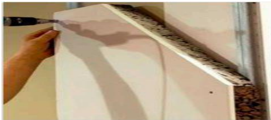
Figure 11: Insulation cork Board glued to gypsum plasterboard in an Internal TICS (GYPTEC, 2012)
