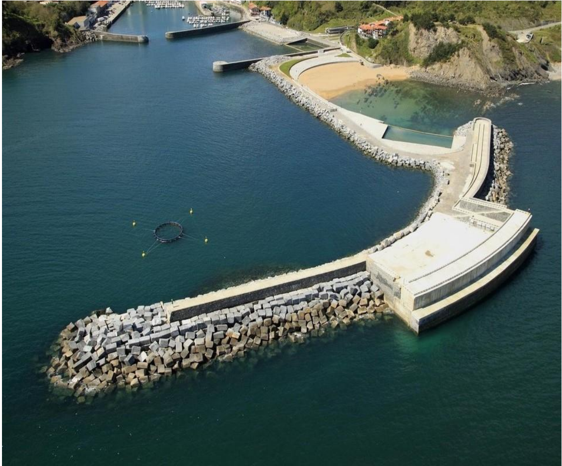
Figure 7: The Mutriku wave energy plant, Spain
